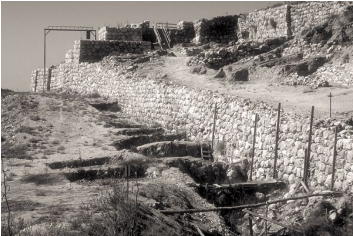
Approach road at Lachish, leading to the gate complex. (Neal and Joel Bierling)
