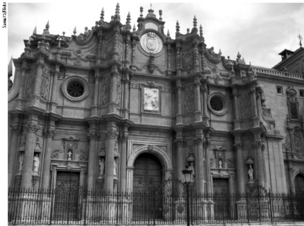
Façade of the Cathedral of Guadix (Granada, Spain).
